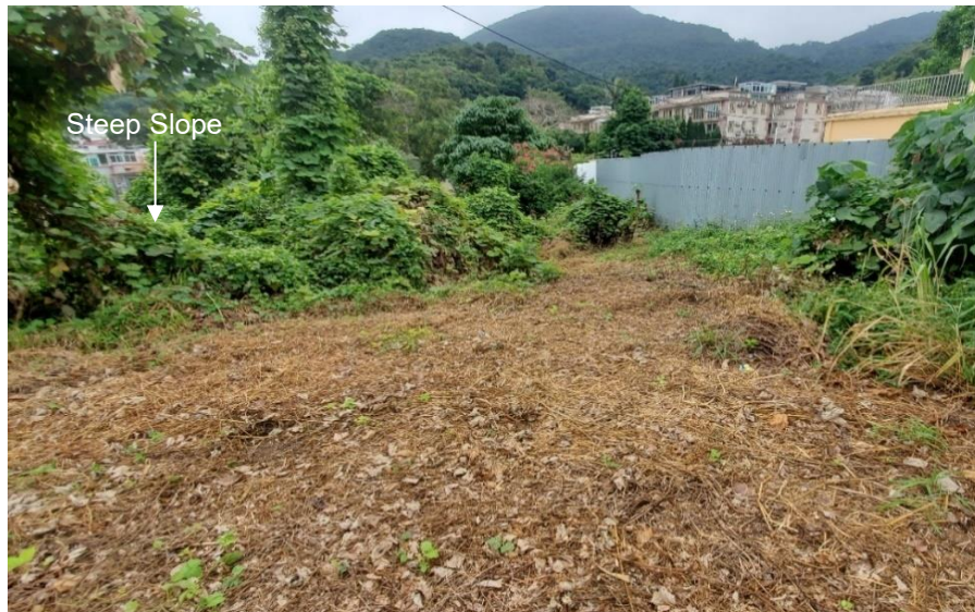
Photo 2.2 Steep Slope in Zone 2 (Facing South)
