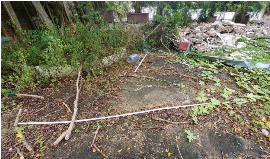
Photo 1.2 Concrete Ground Surface in Zone 1
