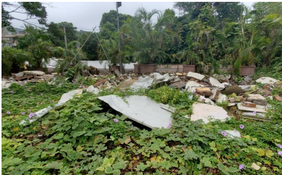
Photo 1.4 Demolished Structures and Construction Waste in Zone 1 (Facing West)
